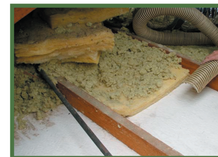
Removing Rockwool and batts
