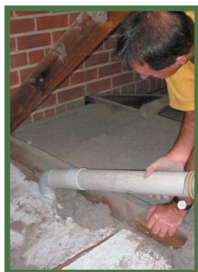
Sucking out cellulose fibre
